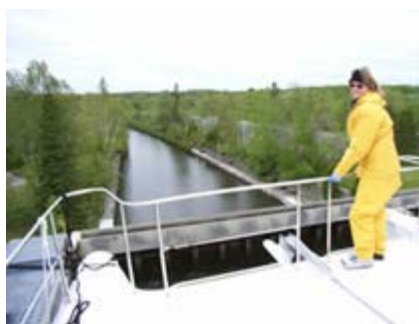
Top of Kirkland Lift Lock at 49 feet
