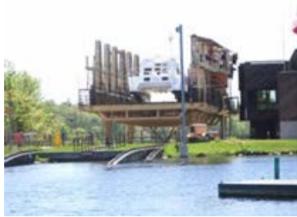
Being lifted on the rail bed
