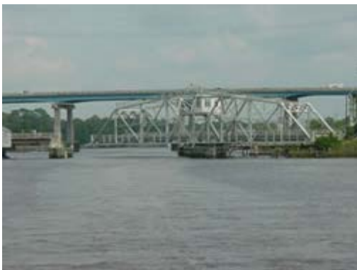
Interesting swing bridge in ICW
